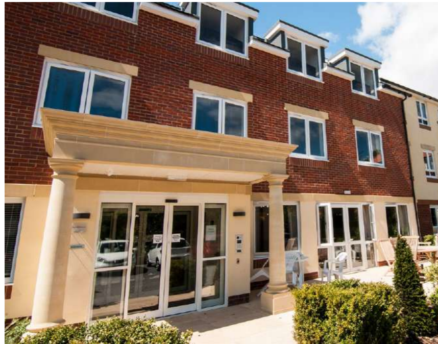
Secure Main Entrance from Parking
